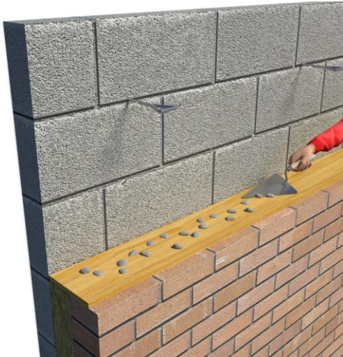
Figure 4 Use of cavity board for clearing off mortar
